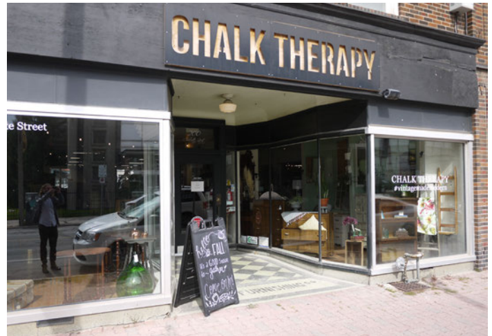
Recessed retail entry in heritage building
