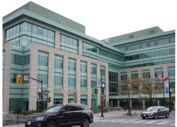
Example of building with screened rooftop mechanical systems
