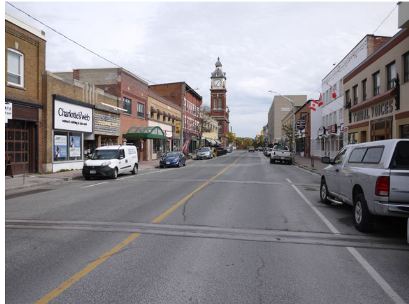
Existing conditions on Charlotte Street east of Aylmer Street
