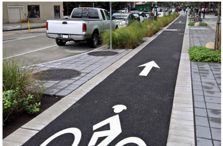
Protected cycle tracks at sidewalk level
