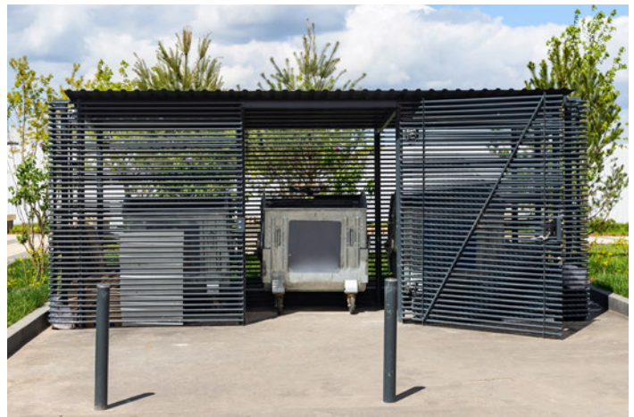
Fully enclosed garbage enclosure
