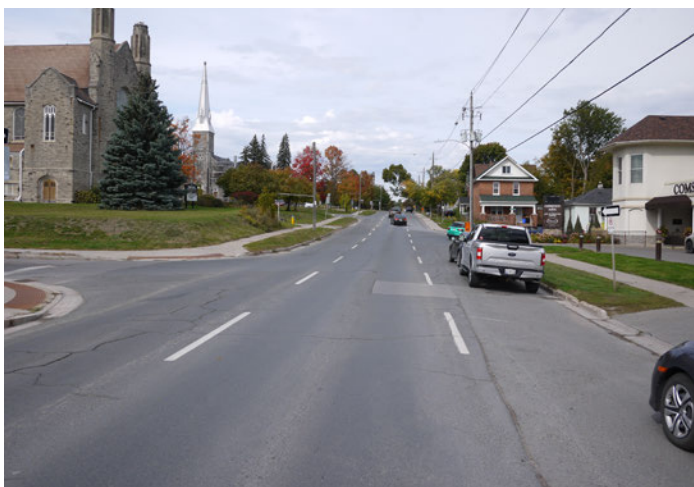
Rubidge Street in the Church Row sub-area of the Downtown Neighbourhood area
