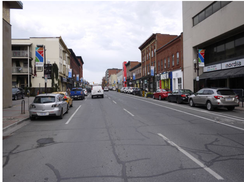
Existing conditions on Water Street
