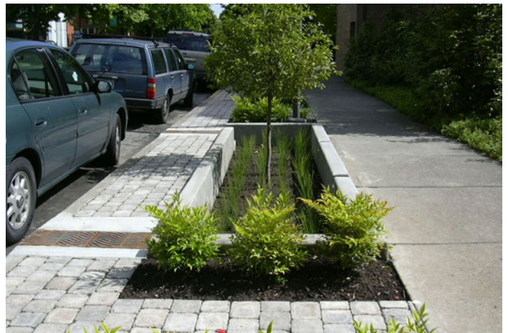
Trees in open planting beds that also function for stormwater management
