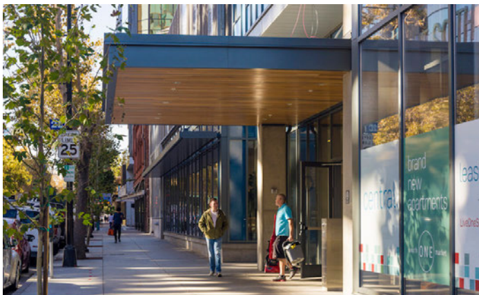
Canopy protecting major building entrance
