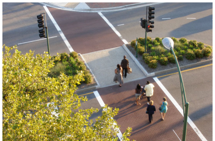
Pedestrian crosswalk defined by special paving and a refuge
