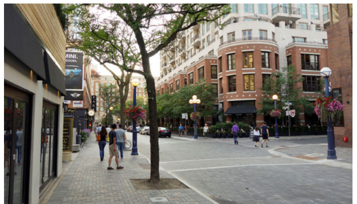
Special paving across sidewalk and road, Yorkville Avenue, Toronto
