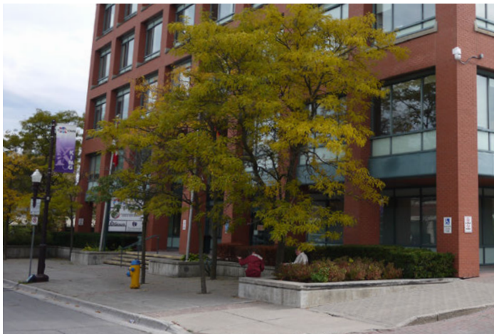
Forecourt of Peterborough Public Health building, King Street
