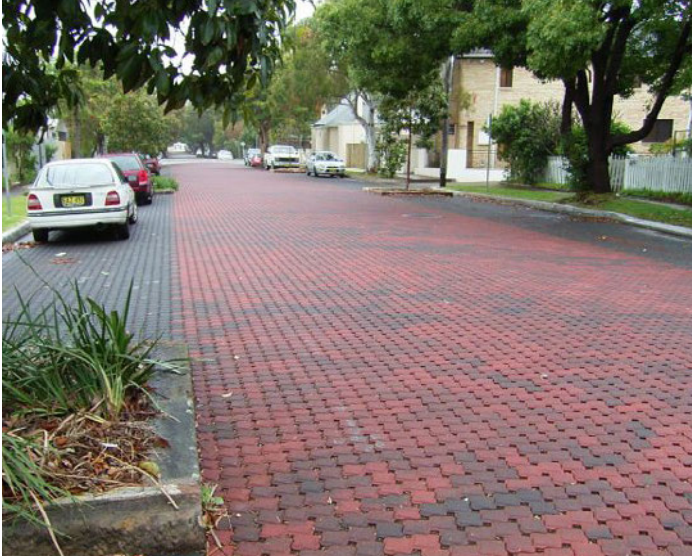
Permeable paving used on a street
