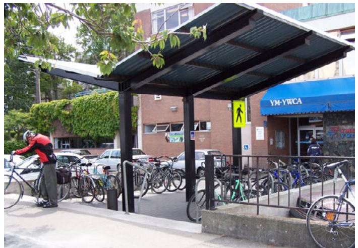
Canopy protecting bicycle parking area
