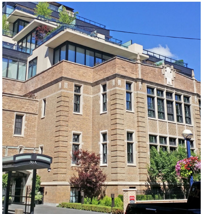
Stepbacks above the heritage building minimize the impacts of increased height on the heritage streetscape
