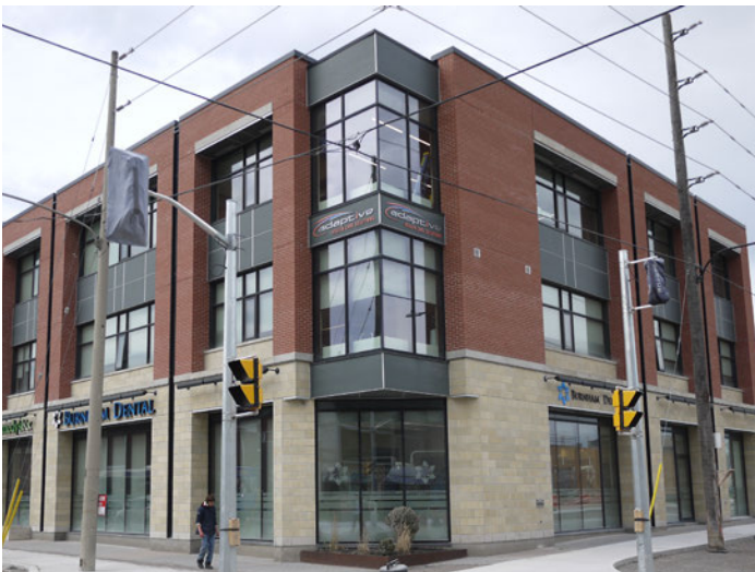
Corner articulation in a mixed use building
