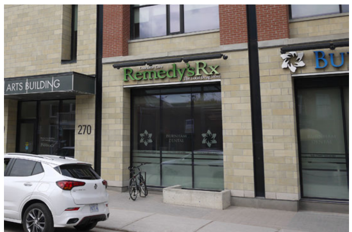
High ground floors allow more flexible and adaptable future uses
