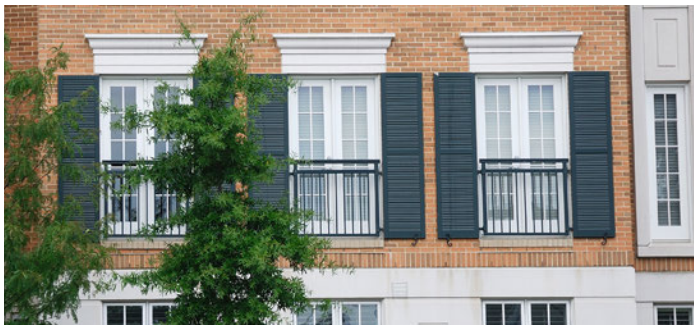
Consistent detailing of new construction in traditional style
