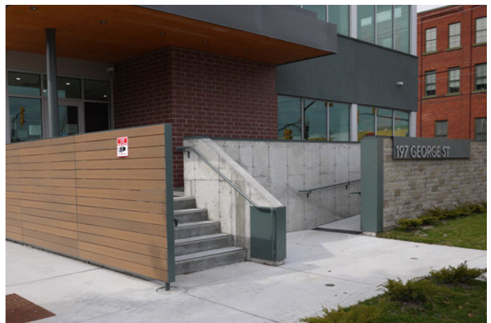
Ramp does not extend into the public right-of-way
