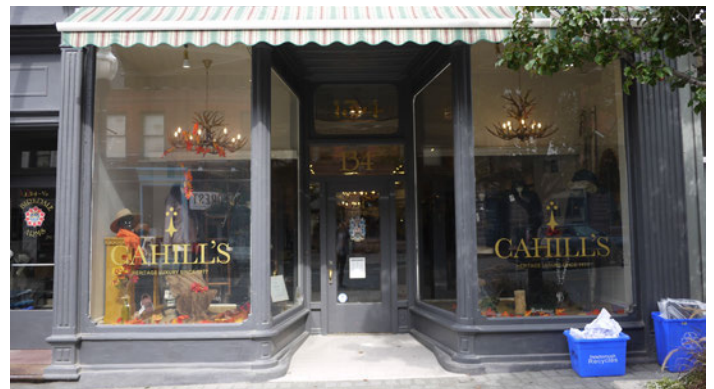
Barrier-free recessed retail entrance
