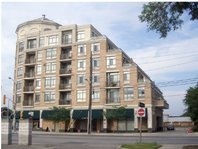
Building showing application of 45 degree angular plane from a side/rear property line
