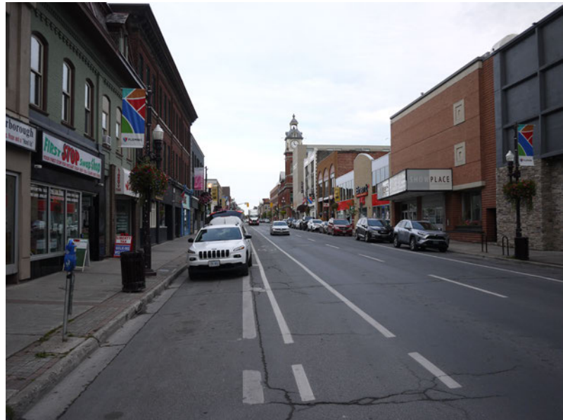
Existing conditions on George Street North
