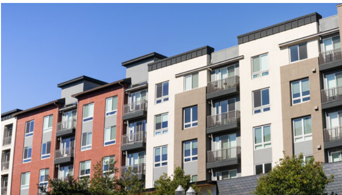
Use of material, colour, variation of setback and roof line
