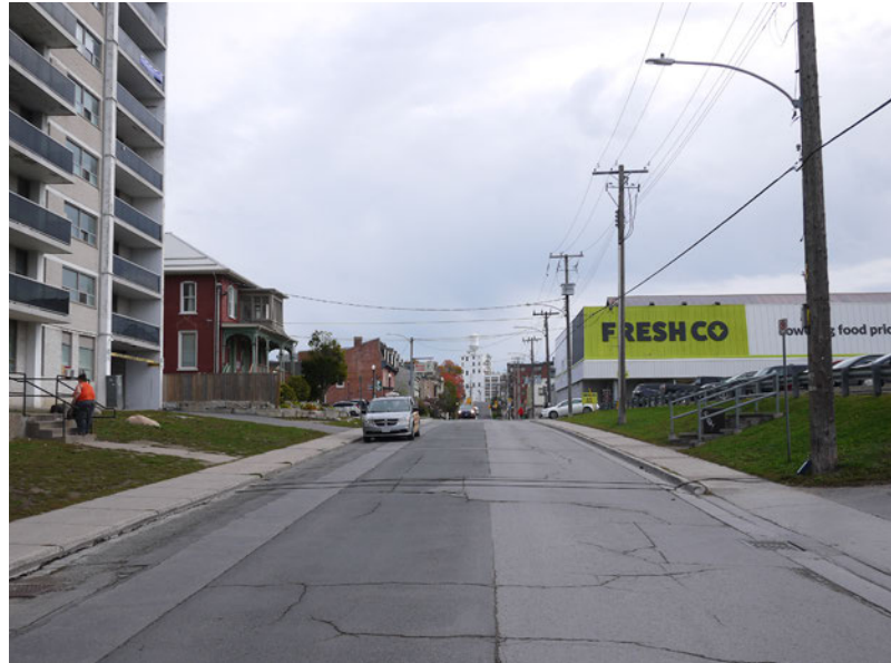
Existing conditions on Brock Street east of Aylmer Street
