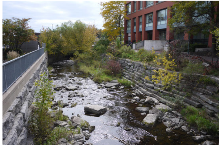
Exposed Jackson Creek south of King Street
