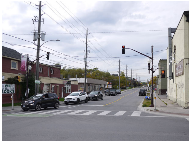
Existing conditions on Sherbrooke Street
