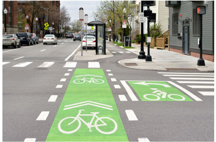
Bike box and bike lane markings crossing an intersection
